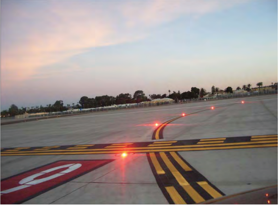
FIGURE 2-1-12 Runway Entrance Lights
