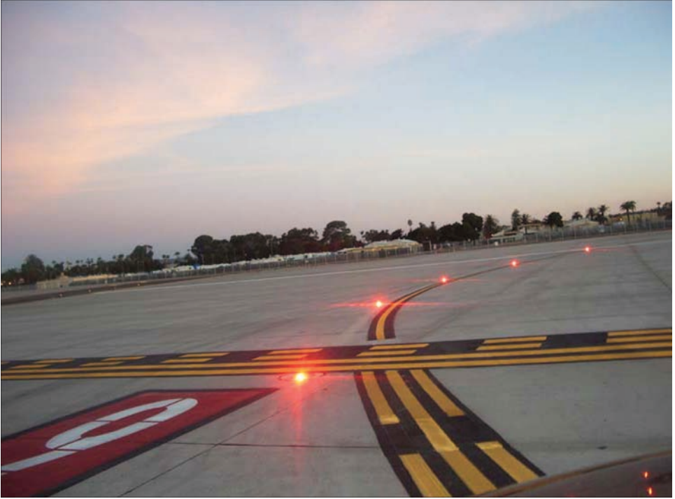
FIGURE 2-1-12 Runway Entrance Lights
