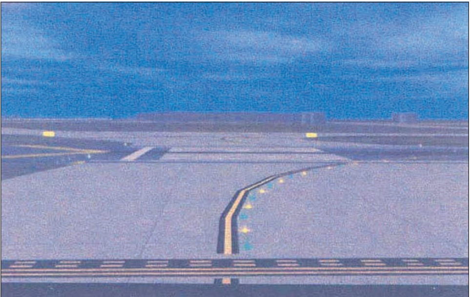
FIGURE 2-1-14 Taxiway Lead-On Light Configuration
