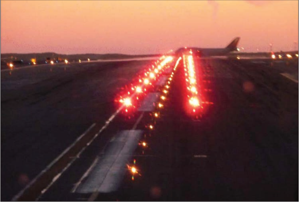
FIGURE 2-1-13 Takeoff Hold Lights
